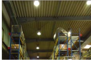
Photo 2. installation of LED in hall 8
