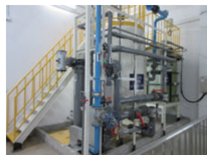
At Kubota Agricultural Machinery (Suzhou) Co., Ltd. (China), we installed recycling treatment equipment for reusing wastewater from processes throughout the entire plant, and this has realized zero emissions of process wastewater. In 2020, we reduced the amount of water usage by 140,000 m 3 .
