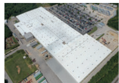
Installation on Building No.2 (2020)
