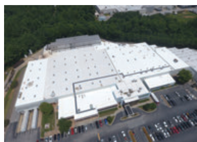
Installation on Building No.1 (2019)
