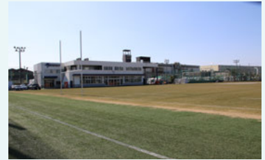
Rugby field on which water granulated slag is used
