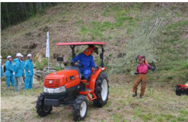
Clearing bamboo on a slope
