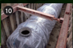
10 Earthquake resistant reservoirs: used to ensure the supply of drinking water when water services are halted due to an earthquake or other disaster.
