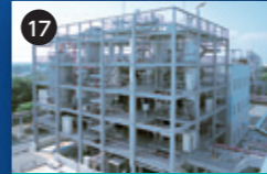
17 Sewage sludge incinerators: plants used to incinerate or melt sludge produced during sewage treatment
