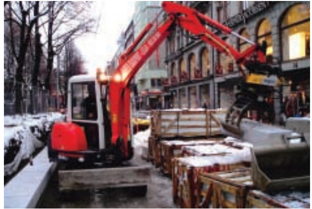
Work in progress using a miniature backhoe (Overseas)
