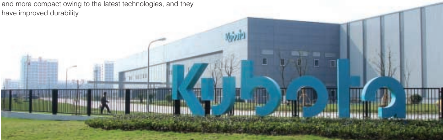
New KAMS plant completed last year
