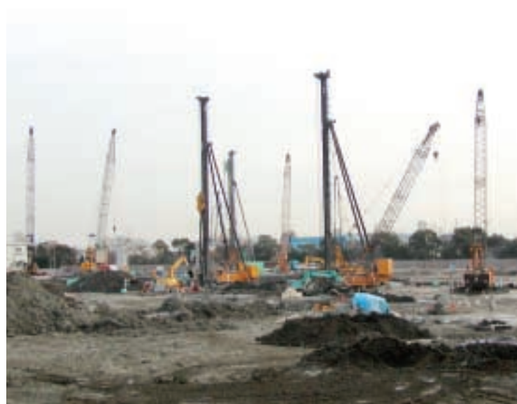
Piling construction site
