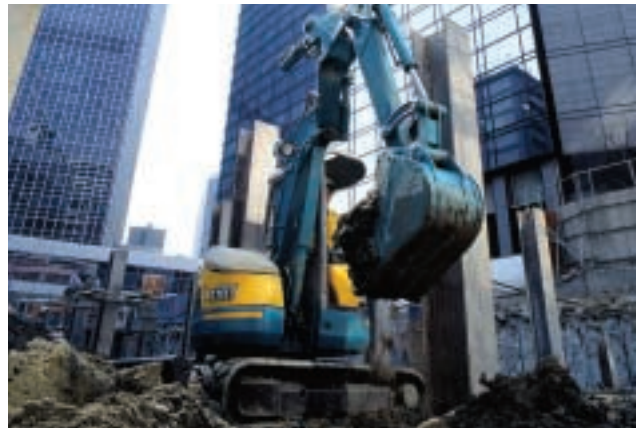
Work in progress using a miniature backhoe (Japan)
