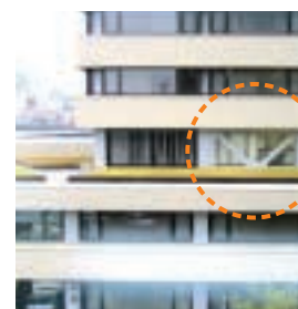
Head Office Building No. 2 reinforced for earthquake-resistant
