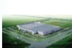
*19 Image of the completed plant
