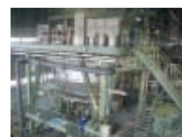
*21 Processing capacity 16 ton/day
