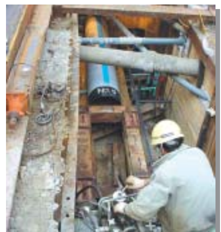
The construction of PN-type propulsive pipes is under way
