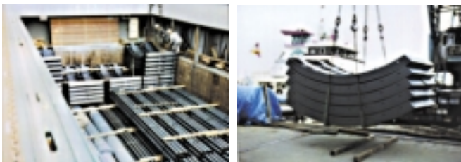
Loading segments in the ship
