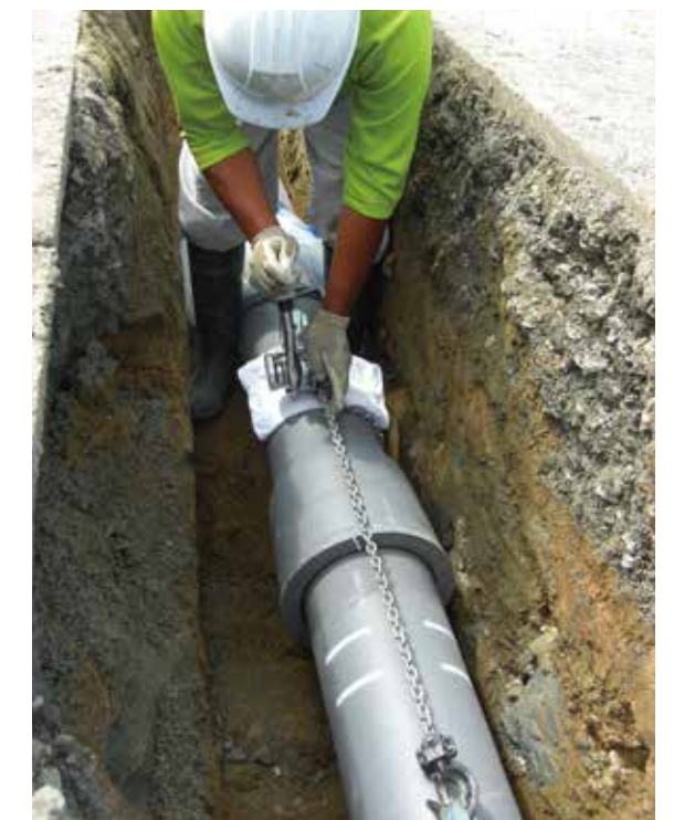
Joining work of push-on joint (GX-type)
