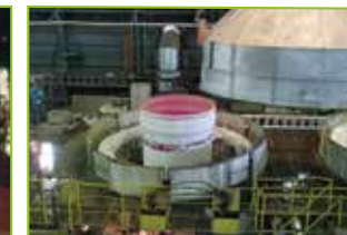
middle and large diameter pipes (Hanshin Plant)
