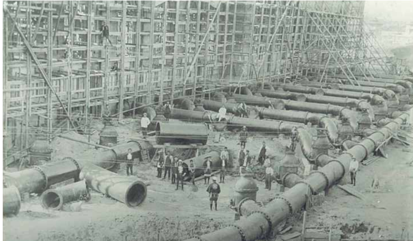
KUBOTA 48 inch pipes & valves, Osaka city, Japan. (1914)
