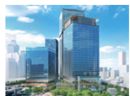
Planned final design of GRAND GREEN OSAKA Park Tower (Source: GRAND GREEN OSAKA Developer)
