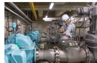
Inspection of water purification plants
