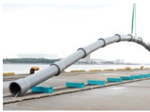
Installed earthquake-resistant ductile iron pipes for the first time in the U.S.
