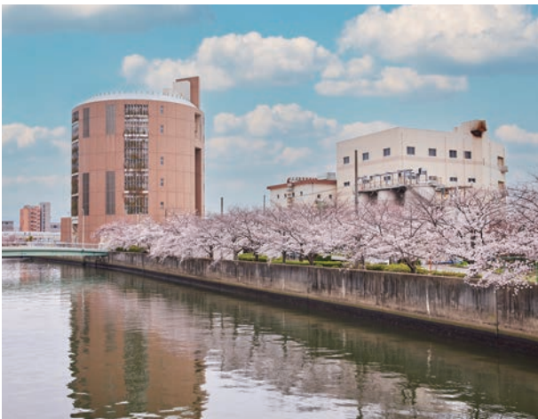
Nakahama Sewage Treatment Plant in Osaka
