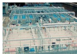
At the Nakahama Sewage Treatment Plant, waste water is treated using membrane bioreactor (MBR) treatment.
