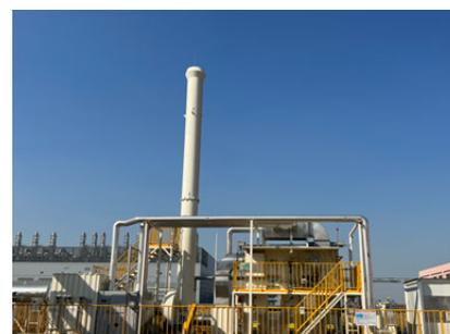
Kubota Engine (WUXI) Co., Ltd. (China) has installed a regenerative thermal oxidizer (RTO) and is working to reduce its VOC emissions.
