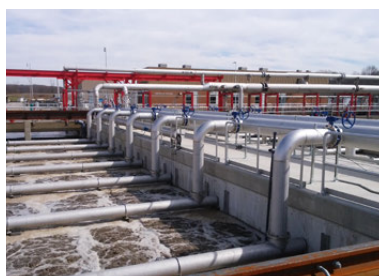
Submerged membranes can also be used to recycle wastewater
