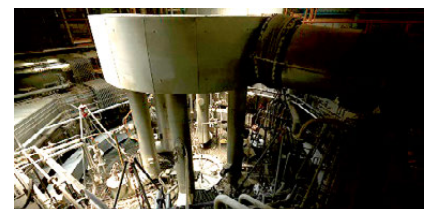
Rotary-type surface melting furnace that can liquefy residue and ash, turn it into slag, and reuse it as a resource
