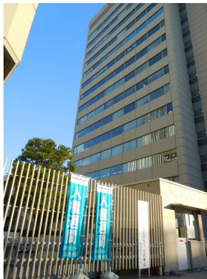
Installation of banners (headquarters)
