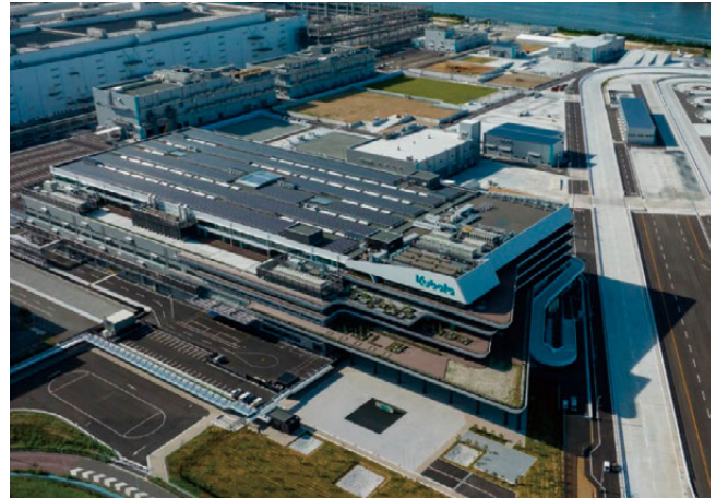
Solar panels capable of generating 1,566 kW of power were installed at the Kubota Global Institute of Technology (Japan), a facility that opened in September 2022.
