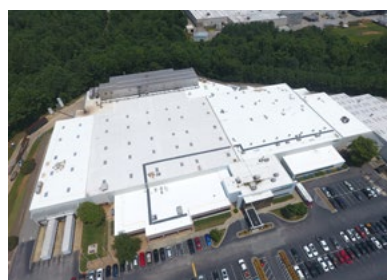
Installation on Building No.1 (2019)
