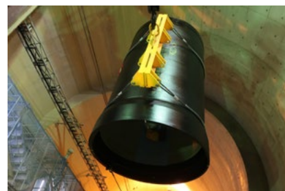
Earthquake-resistant ductile iron pipe Nominal diameter 1500 – 2600 US type (R type)
