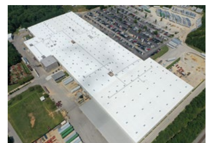
Installation on Building No.2 (2020)
