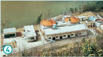
Night soil treatment plant in Miyoshi, Hiroshima, the first project after the Division was formed
