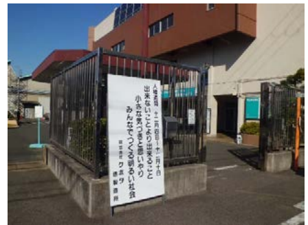
Installation of standing signboards (Sakai Plant)
