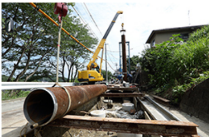
Spiral welded steel pipes (used as foundation piles in a variety of structures, such as bridge foundations, ports, rivers, and building foundations)
