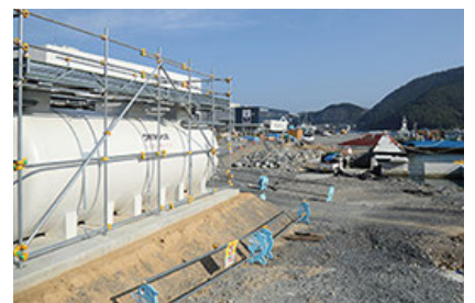
Wastewater treatment tanks (used to process wastewater from temporary housing in regions with insufficient sewage lines)
