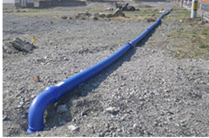
Plastic pipes (used in the restoration and maintenance of lifelines, such as water supplies, sewage lines, and gas lines)
