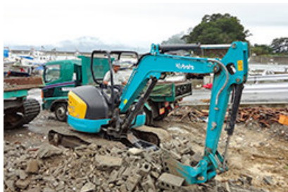
Construction machinery (used for removing debris and various civil engineering work)
