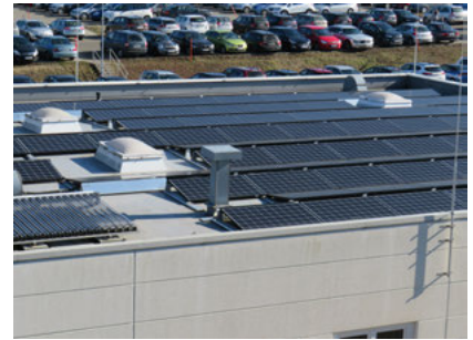
Installation of solar power generation system Kubota Baumaschinen GmbH (Germany)
