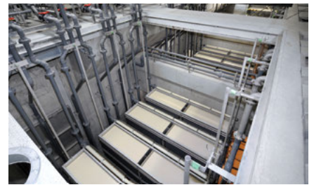
Submerged membranes: used to purify wastewater, including industrial and domestic sewage.
