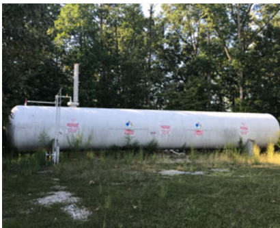
Before and after the removal of plants Kubota Manufacturing of America Corporation (US)
