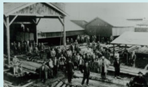
Kubota iron pipe shipping site around 1905
