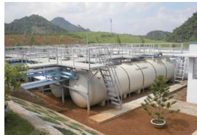
Wastewater treatment plants (Johkasou): used to treat wastewater in areas where there are no sewage lines.
