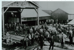
Kubota iron pipe shipping site around 1905
