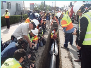
Installing the earthquake-resistant pipe “GENEX®” in Los Angeles
