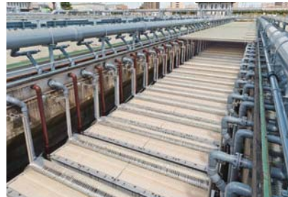
Submerged membranes: used to purify wastewater, including industrial and domestic sewage.
