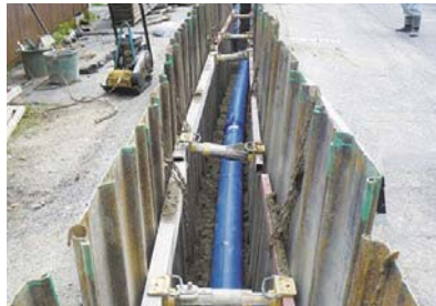
Plastic pipes: used in infrastructure, including water and sewage lines, and gas piping.
