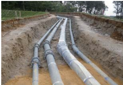
Ductile iron pipes: used in infrastructure, including water and sewage lines, and agricultural water facilities.
