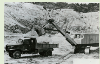
Mechanical power shovel performing loading (KB60 type)
