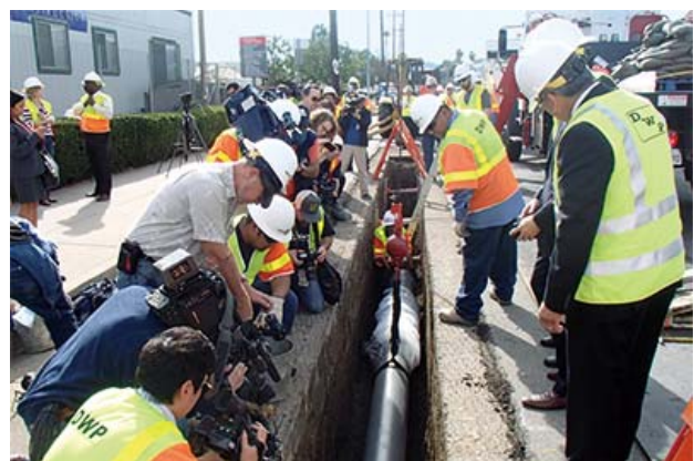
Laying GENEX® earthquake-resistant pipe (Los Angeles, U.S.)
