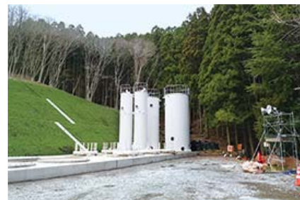
Pre-treatment facility under construction
