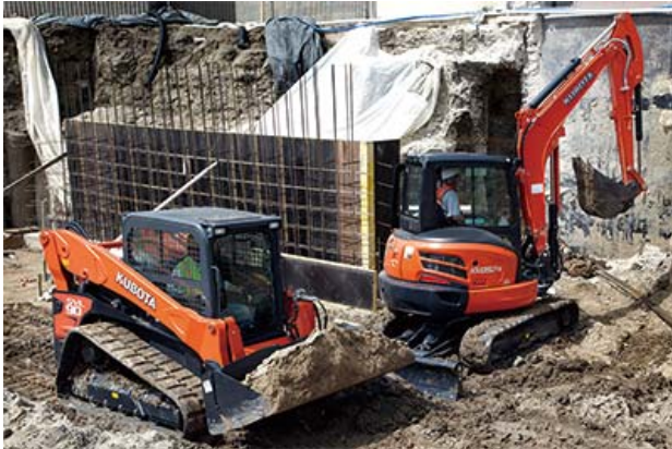
(Left) Compact track loader (Right) Mini excavator
