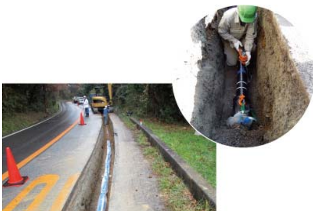
Laying NECS® earthquake-resistant pipe (Nose, Osaka)
