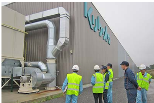
Environmental audit at overseas production site Kubota Farm Machinery Europe S.A.S
