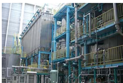
Water treatment plant This is used to purify waste water, including residential and industrial sewage.
