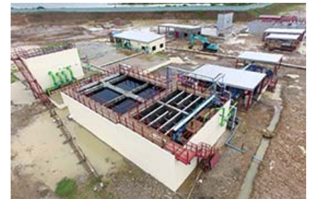
Thilawa Industrial Park Zone A Water Purification Area (Myanmar)
