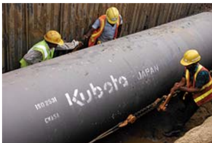
Laying ductile iron pipes (water pipes) (φ1,200 mm) (Bangladesh)
