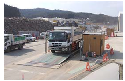
Truck scales Truck cargo, such as debris, is weighed.
