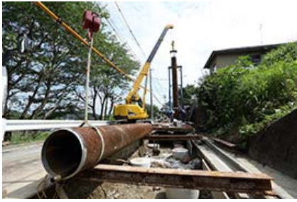
Spiral welded steel pipes This is used as foundation piles in a variety of structures, such as bridge foundations, ports, rivers, and building foundations.
