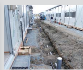
Plastic pipes This is used in the restoration and maintenance of lifelines, such as water supplies, sewage lines, and gas lines.
