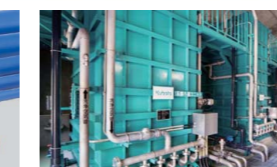
14 Ceramic film: used in the purification process for sources of water, including river water, to create clean drinking water.
