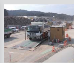
Truck scales Truck cargo, such as debris, is weighed.
