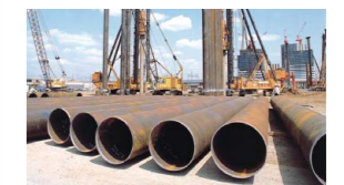
18 Spiral welded steel pipes: used in foundation construction, including for buildings and bridges in addition to harbor and river projects.
