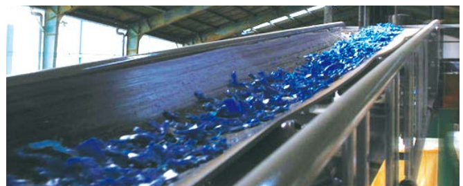
Crushing and recycling plants: used to crush and sort recyclable garbage to enhance its resource value so that it can be reused or turned into raw materials or fuel.
