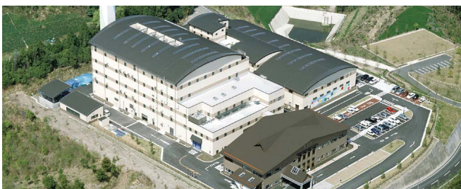
Waste incinerator plants and ash and melting furnace plants: used to incinerate and reduce the volume of municipal waste, as well as to contribute to decarbonization of society by using the large quantity of waste heat to generate electricity.
