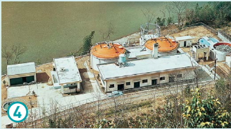
Night soil treatment plant in Miyoshi, Hiroshima, the first project after the Division was formed
