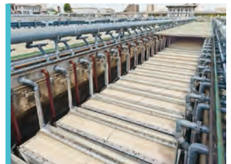
Membrane solutions Used to purify waste water, including industrial and domestic sewage.
