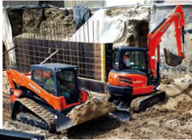
(Left) Compact track loader (Right) Mini excavator
