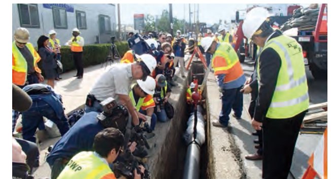
Laying GENEX® earthquake-resistant pipe (Los Angeles, U.S.)
