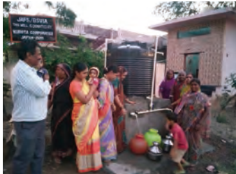
Supporting well construction in India
