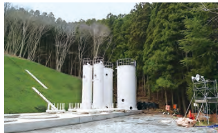
Pre-treatment facility under construction
