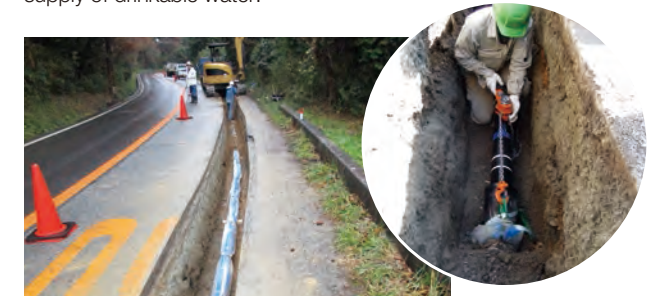
Laying NECS® earthquake-resistant pipe (Nose, Osaka)
