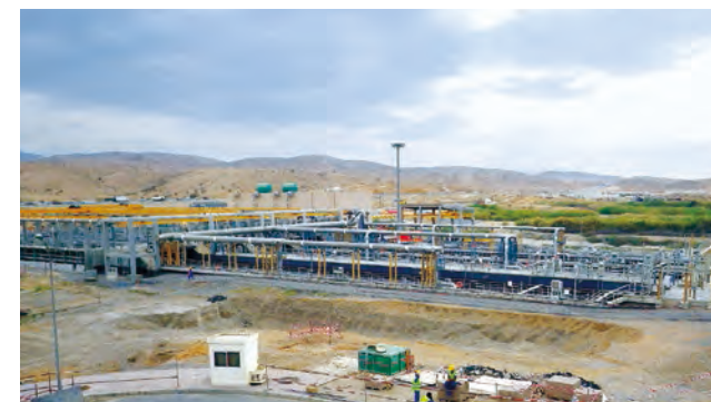
Al Ansab Sewage Treatment Plant (Oman)
