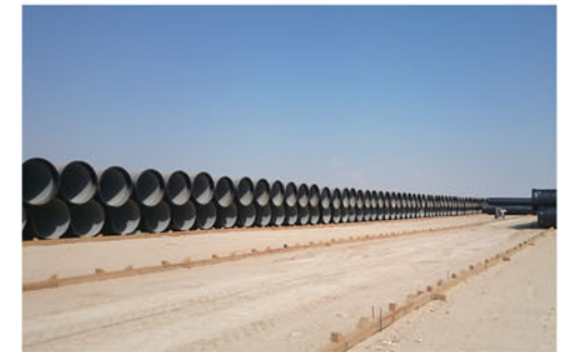
Ductile iron pipe used for water pipeline
