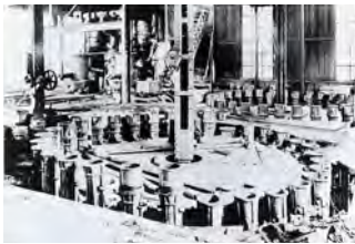
Cast iron pipes for water supply (1893)
