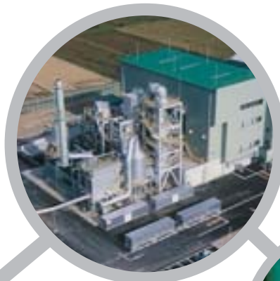
Industrial waste processing facility
