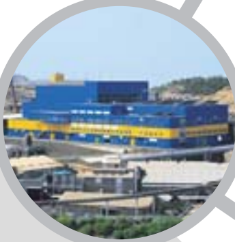
Intermediate treatment plant
