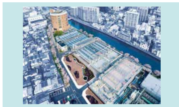
Fig. 1 Nakahama Sewage Treatment Plant after Reconstruction
