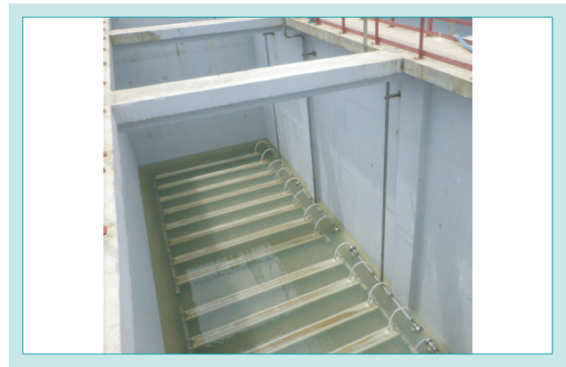
Fig. 13 K-membrane Installed in the Thilawa SEZ Zone
