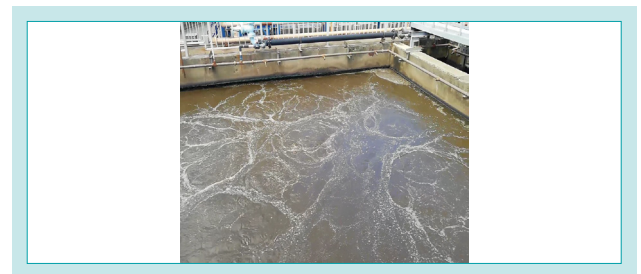
Fig. 5 View of Aeration in the Field (August 2018)
