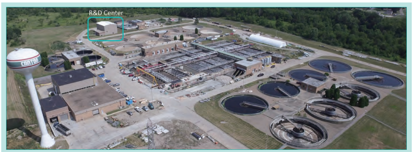
Fig. 2 Overview of the Canton Water Reclamation Facility and Location of the R&D Center
