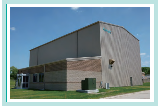
Fig. 3 Outside View of the Facility
